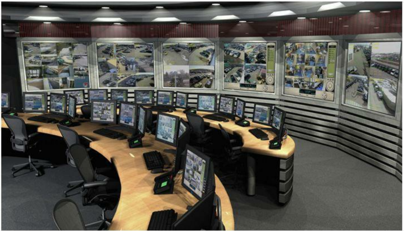
Figure 10.17 - The Central Center, also known as the Security Console Center, security control center or dispatch center is an area that serves as a central monitoring and assessment space for access control, CCTV, and intrusion detection systems (Courtesy of Bosch Security Systems)
