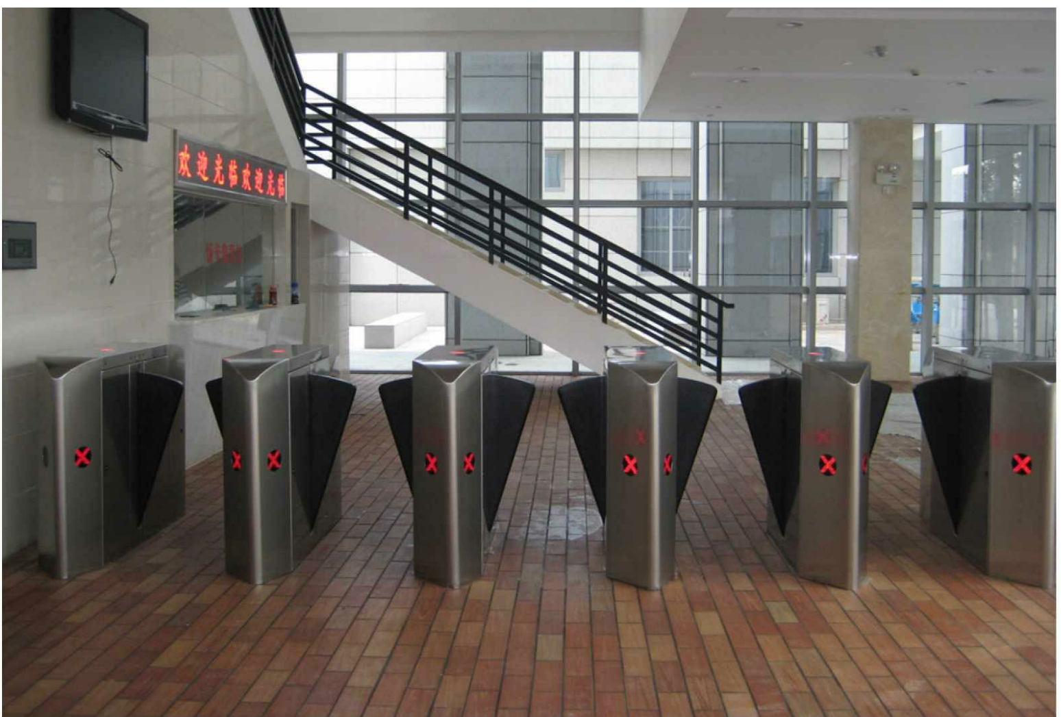
Figure 10.25 - A higher end turnstile is an optical turnstile, which is designed to provide a secure access control in the lobby of a busy building (Courtesy of Bosch Security Systems)
