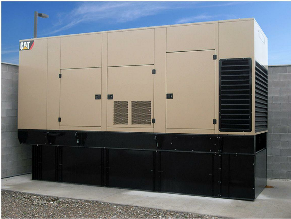
Figure 10.36 - A Backup Generator is activated automatically in the event of a utility failure by the transfer switch. (Courtesy of Bosch Security Systems)
