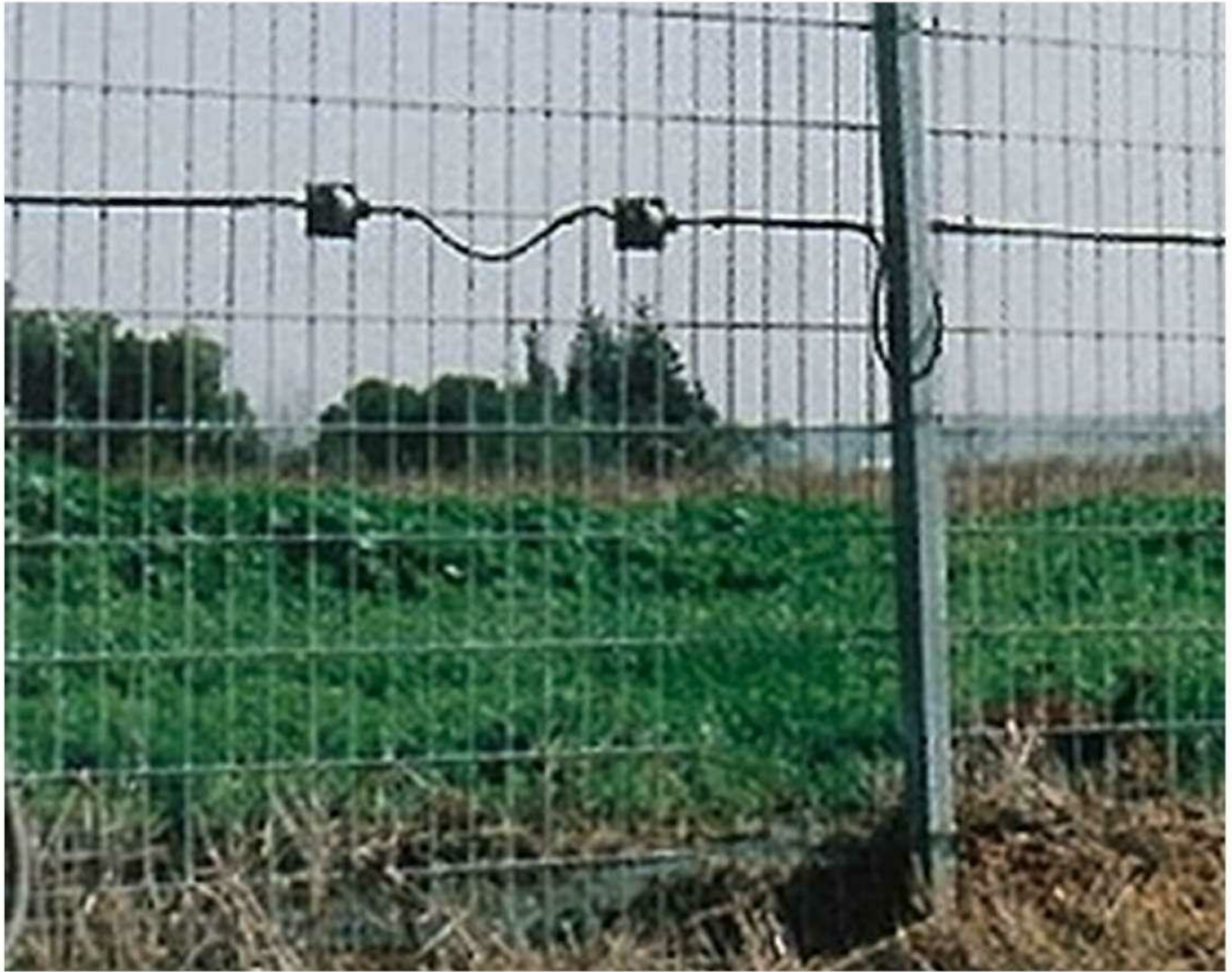
Figure 10.10 - Coaxial Strain-Sensitive cable (Courtesy of Bosch Security Systems)
