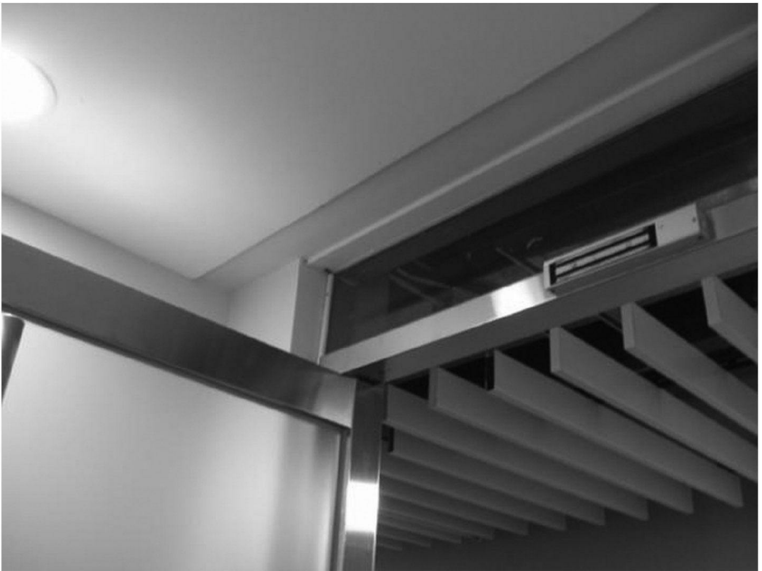
Figure 10.22 - Magnetic Lock (Courtesy of Bosch Security Systems)
