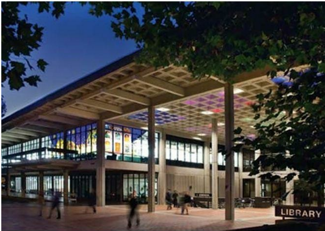
Figure 10.4 - Building designed with crime prevention in mind
